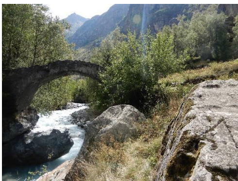
8051: the bridge from downstream
