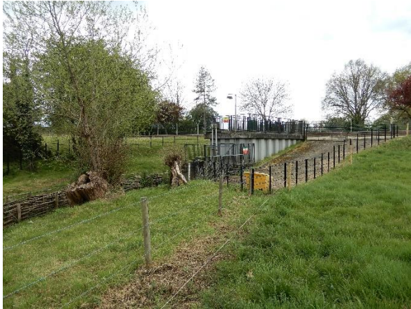
4319: culvert under George 5 th Avenue
