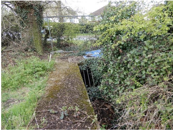
4304: culvert under the main road
