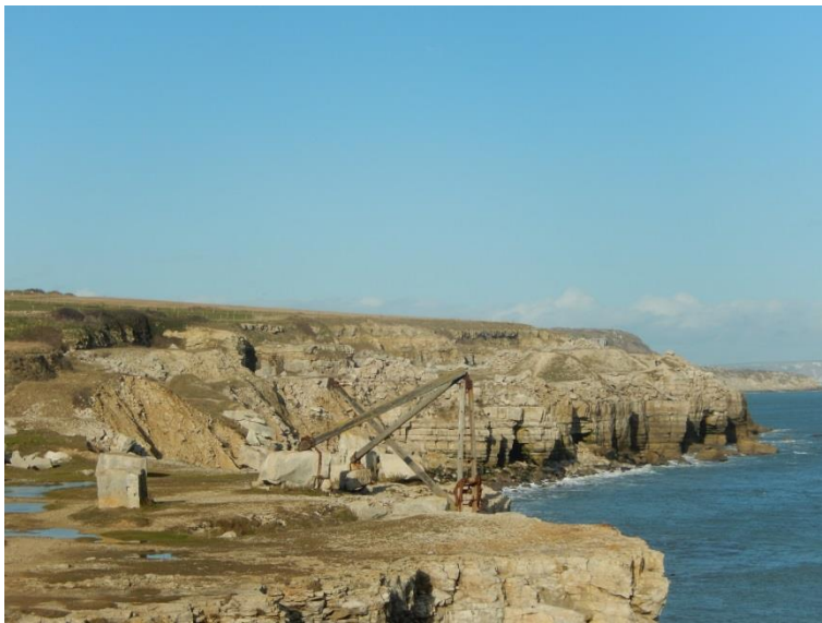
The hoist for loading the rocks
