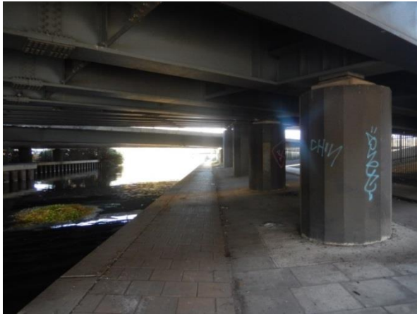
Photo7430: under the Lee Valley Viaduct
