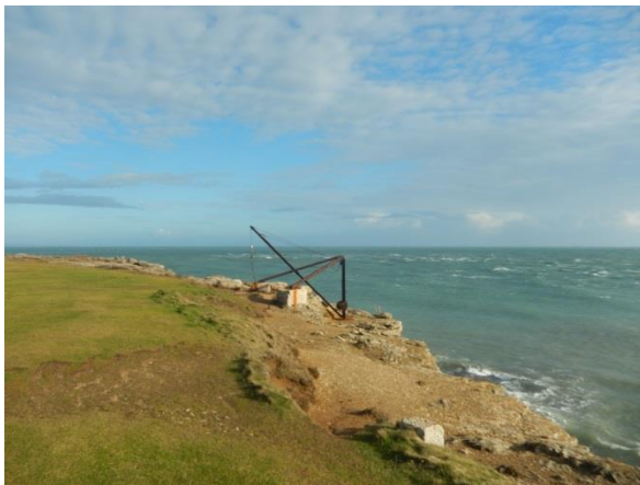
There were several of these hoists
