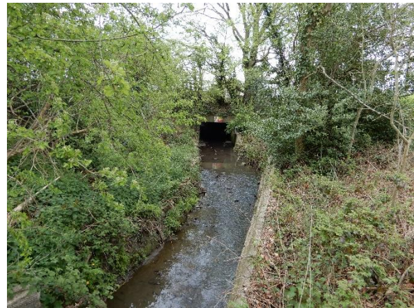
4320: from the footbridge towards the culvert
