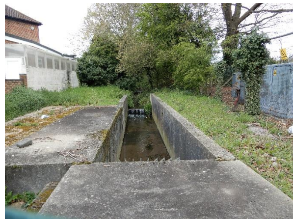
4305: culvert under the roundabout
