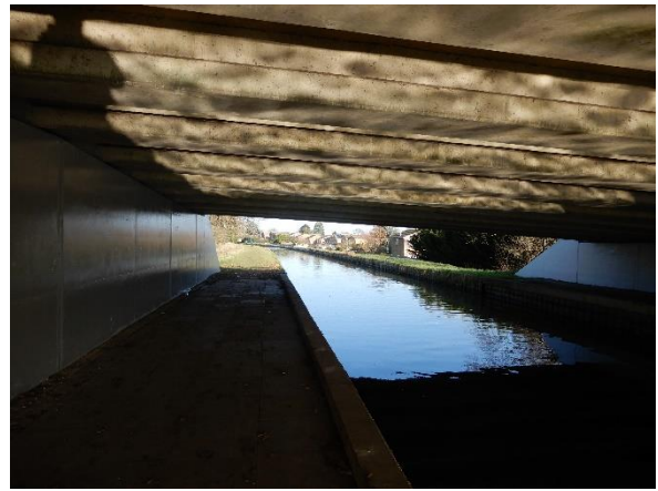
5846: under the A10
