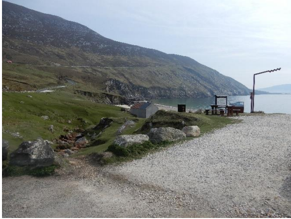
6608: spot is by the bent pole
